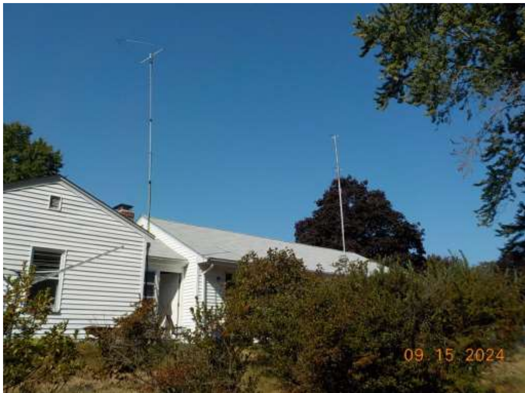
Above: Figure 1 – On the left is the PAR Electronics OA-50 omnidirectional antenna and on the right are the two stacked and phased OA-144 omnidirectional antennas at W1NIV's station.
