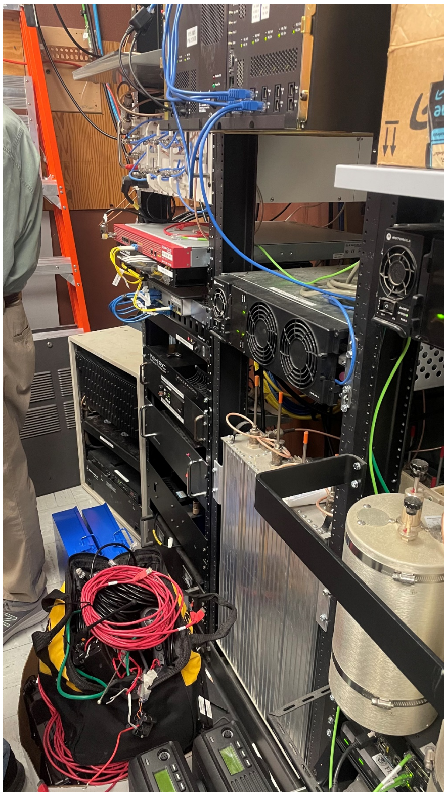
Figure 19-Shared repeater room. The FARA repeater enclosure (white) is the one on the floor next to the orange ladder. The repeater is the thin component near the bottom of the cabinet. The component (with the grill) at the top of the enclosure is an amplifier.
