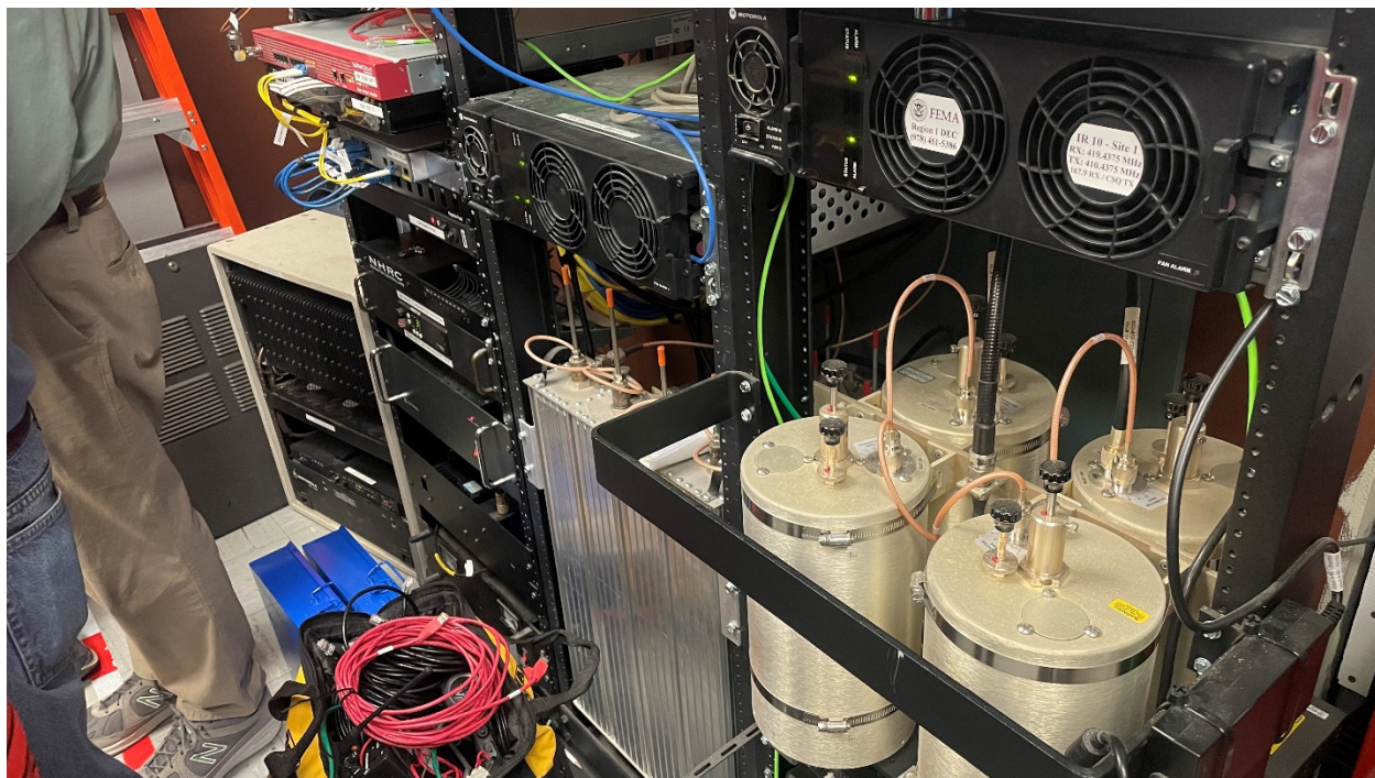
Figure 20-Shared repeater room (continued). The repeater puts out one Watt and the amplifier steps it up to 110 Watts. The output ends up being about 80 Watts.
